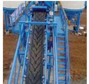
Aggregate weighing and transfer to mixer by belt (No skip bucket)
