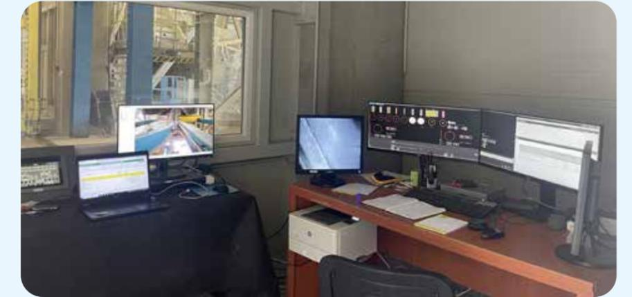
SIMEM@TIC is the automation control system with a friendly interface which displays all essential plant operation information. A full process sequence view (loading, weighing, recipe, discharge, washing, production listing, pending orders) with self-adjusting software for a predictable and repeatable outcome. All production data is recorded and stored in SQL database format providing detailed record of concrete production.
